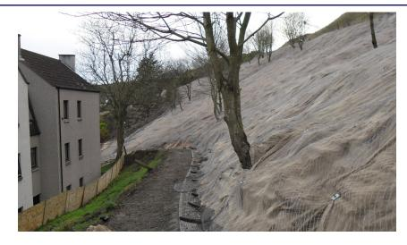
The length and steepness of the slope, the restricted access to the base of the slope together with the large number and length of soil nails meant that conventional soil nailing equipment including excavator mounted feed beams or rope access equipment was not suitable for this location and we established an innovative system of tracked, air powered rotary percussive drilling rigs secured and hauled by winches which were set up on the closed Bervie Braes road.
